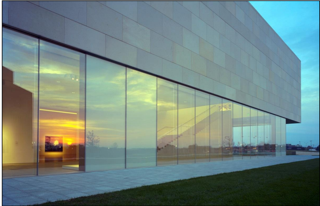
Façade: Local limestone with glazing | photo courtesy of KSWA
